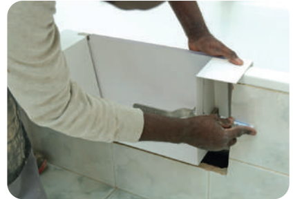
Adaptation based on the thickness of the tub
